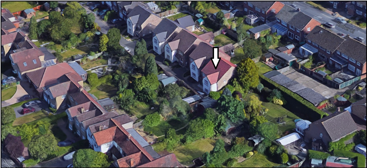
Fig. 1. Aerial view of site.
